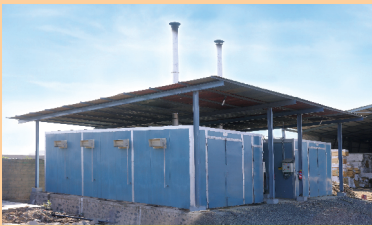
FHAT Plant as Per ISPM-15 Norms. Made from GI 18smg Sheet
